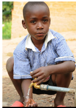
NEW WATER TAP AT SCHOOL, SWS UGANDA
