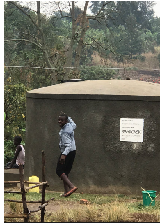
RAINWATER TANK, SWS UGANDA
